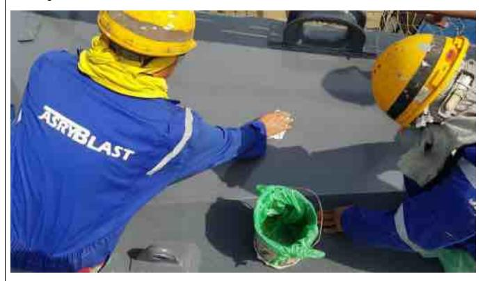
Removing the back film with a pen knife.
