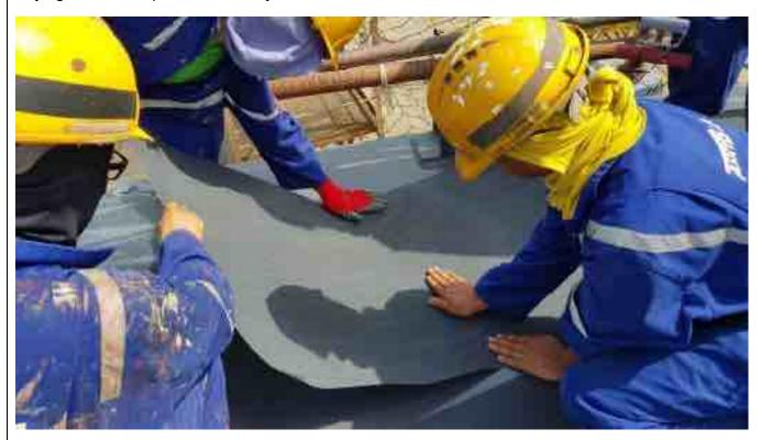
Rolling the Silvagrip panel with a heavy roller. A hand roller can also be used.
